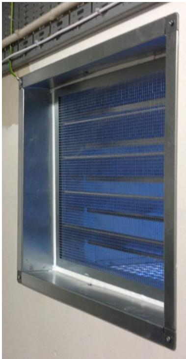
Fig. 7: Mounted backdraught damper in wall
