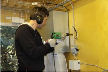
2. If old sheet metal is in the way for the damper's placement, this must be cut away. Brush off any metal shavings that can fall into the fan inlet.
