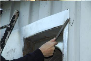
3. Install the damper with self-tapping screws. Seal with silicone sealant between damper and wall.
