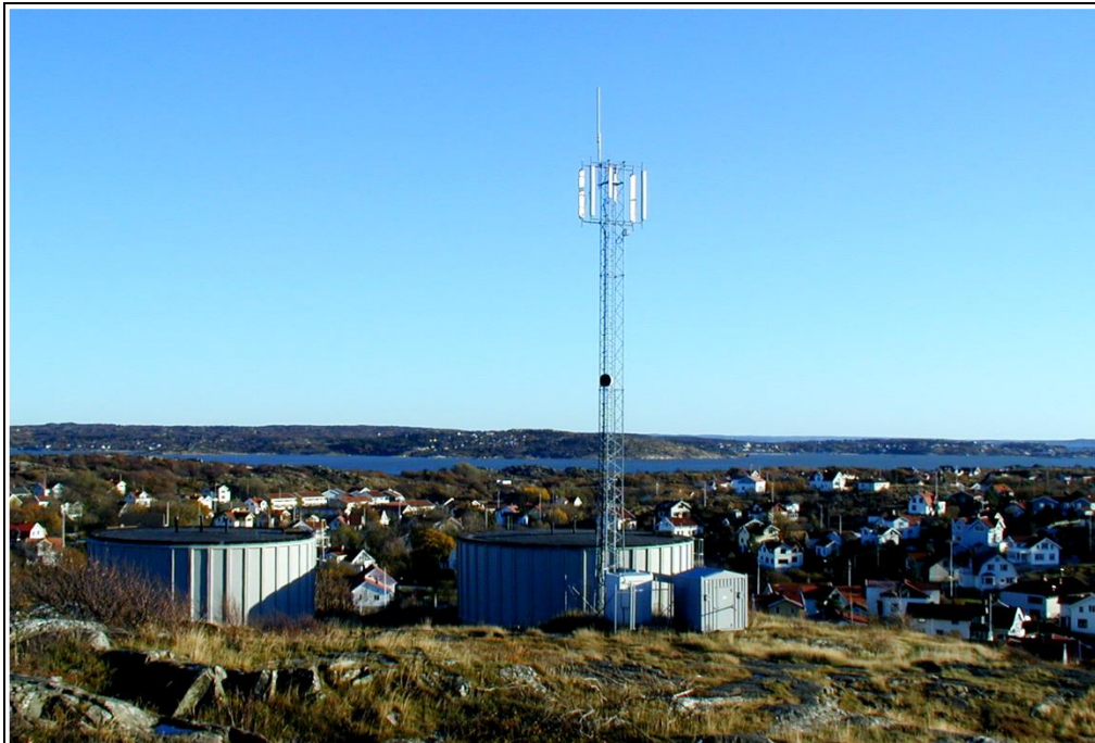
Typical telecom site with FreeCooling at Björkö, in Gothenburgs northern archipelago
