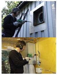
2. If old sheet metal is in the way for the damper's placement, this must be cut away. Brush off any metal shavings that can fall into the fan inlet.
