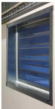
Fig. 7: Mounted backdraught damper in wall
