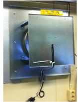
Fig 4: Connection plate with fan (DeltaMaster 2, 6L & 8)
