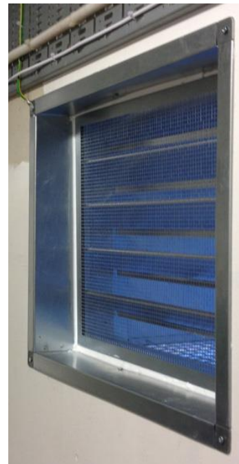
Fig. 5: Backdraught damper mounted in wall
