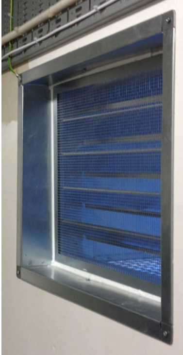
Fig. 7: Mounted backdraught damper in wall
