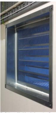
Fig. 7: Mounted backdraught damper in wall
