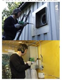
2. If old sheet metal is in the way for the damper's placement, this must be cut away. Brush off any metal shavings that can fall into the fan inlet.
