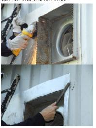
Install the damper with self-tapping screws. Seal with silicone sealant between damper and wall.
