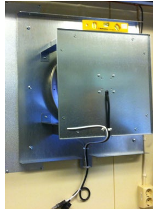
Fig 4: Connection plate with fan (DeltaMaster 2, 6L & 8)
