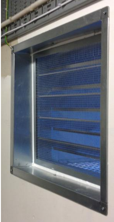
Fig. 7: Mounted backdraught damper in wall
