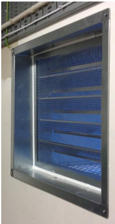
Fig. 7: Mounted backdraught damper in wall
