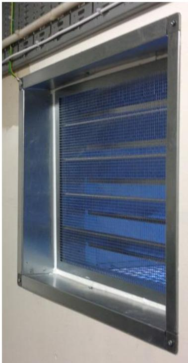
Fig. 7: Mounted backdraught damper in wall
